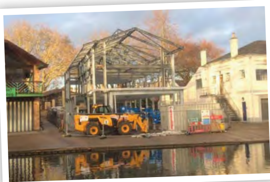
Our boathouse being constructed in May 2019
